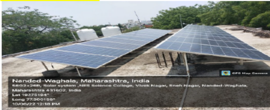
Installed Rooftop Solar Power generation plant of Capacity 5KW in the campus.
